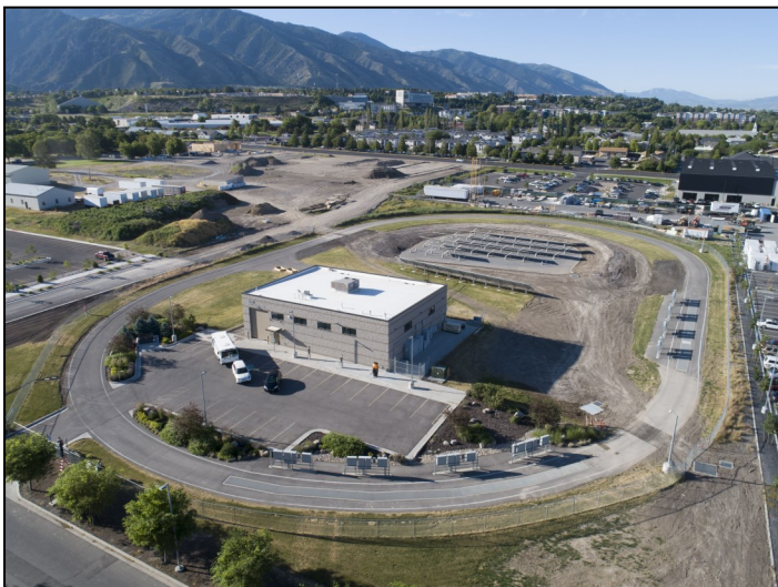
Electric Vehicle and Roadway (EVR) Research Facility at Utah State University
